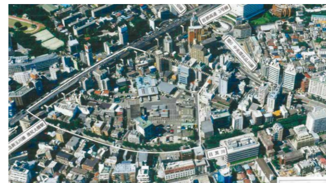
Ohashi Junction site (before construction) Source: Bureau of Urban Development, Tokyo Metropolitan Government.
