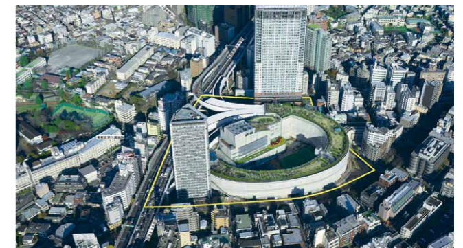
Ohashi Junction site (after construction) Source: Bureau of Urban Development, Tokyo Metropolitan Government.
