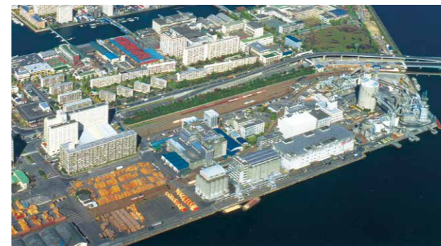
Site of Harumi Island Triton Square (before construction) Source: Harumi Corporation.
