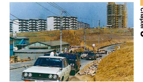
Circa 1971 Construction of housing developments in progress Source: Suwa/Nagayama danchi no ima, mukashi (Suwa/Nagayama housing development today and yesterday), documents donated by the Urban Renaissance Agency. From the collection of the Tama City Cultural Foundation.
