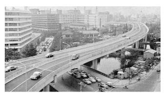
Construction of grade separated roads (the latter half of the 1960s) Construction of the Metropolitan Expressway through grade separation was widely advanced in locations through the city in order to put an end to the severe congestion on Tokyo's roads and make traffic smoother. Source: Kajima Corporation.
