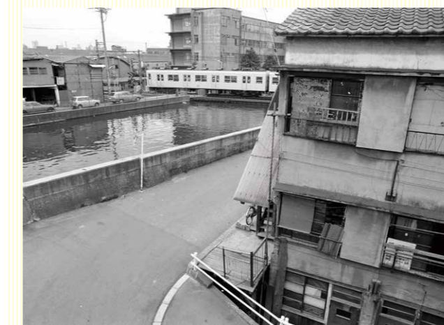
A home positioned lower than the surface of the river due to ground subsidence (1973)
