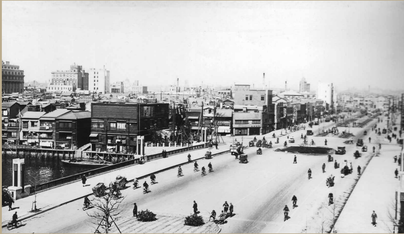
Source: "Reconstruction Work," published in 1930 by the City of Tokyo. From the collection of the Goto Shinpei Memorial Museum. View of the reconstructed city of Tokyo following the Great Kanto Earthquake: Showa-dori Avenue in the area of Edobashi Bridge. Shinpei Goto's reconstruction plan was a colossal project, which saw a century ahead into Japan's future.
