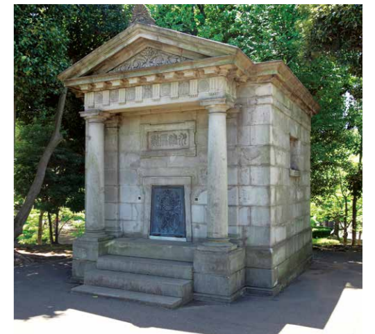
Nihon Suijun-genten Hyoko (Storage for Japanese datum of leveling) Designed under Shichijiro Satachi, this stores the datum of leveling, which was built within the grounds of the General Staff Office (currently Nagatacho, Chiyoda-ku) as the reference in determining elevations in Japan. It is still used as a public structure.
