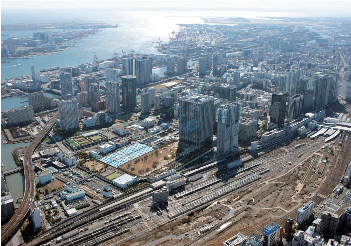
Shibaura Water Reclamation Center (Photo by Bureau of Sewerage TMG)
