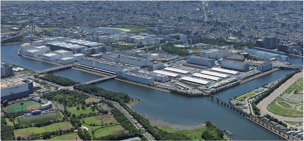
South distribution business complex (Provided by Japan Motor Terminal Co., Ltd.)
